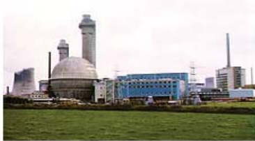
Calder Hall nuclear power station
