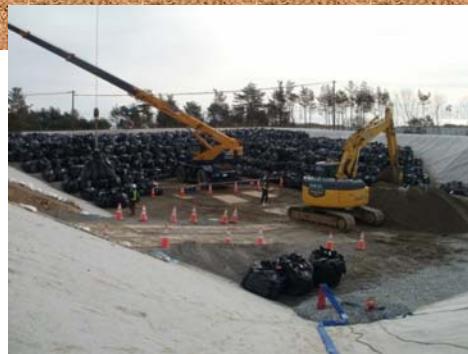
Temporary storage under construction
