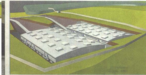
DECOMMISSIONING: low-level waste from the plant will be packed in barrels and then buried in six large vaults. Main picture: Gordon Terris
