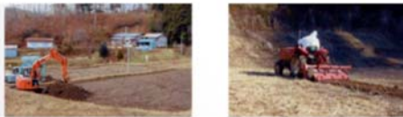
Removal and deep plowing
