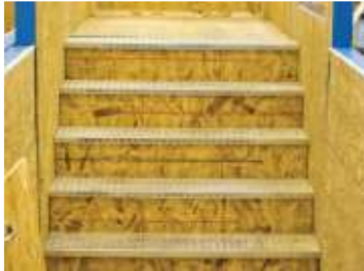
(a) Stairs, landing area
