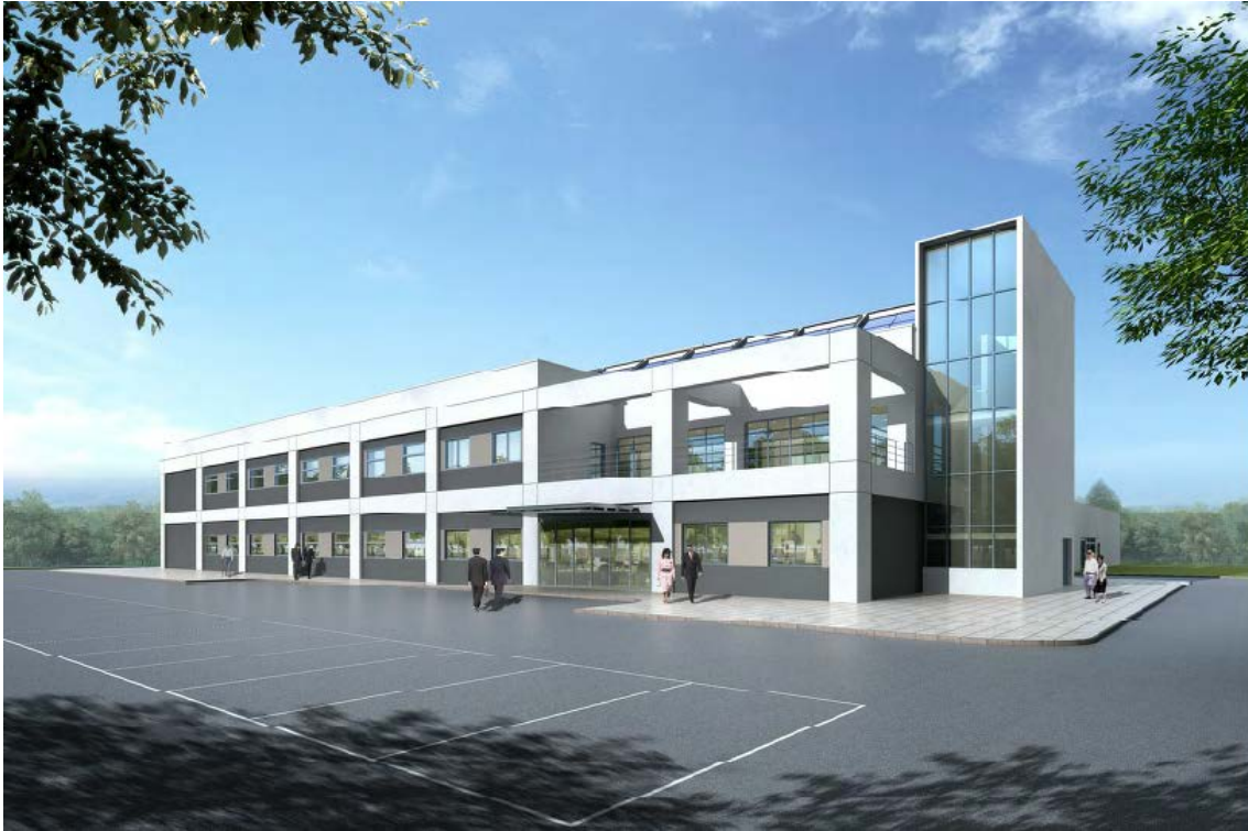
Image of research building being constructed in Minamisoma City*
