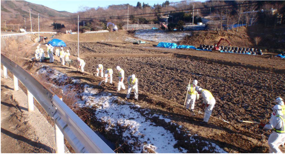
Photograph of decontamination work for farms. The workers are stripping soil at top surface region.
