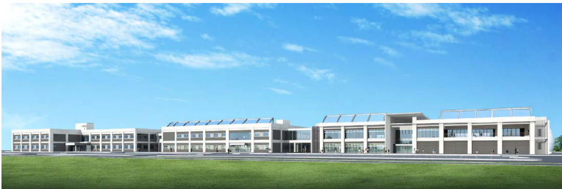
Image of research and exchange building being constructed in Miharu Town*
