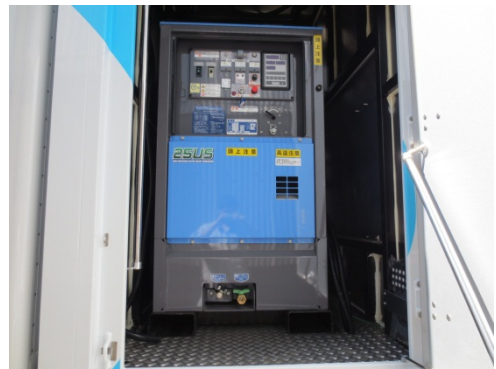
The generator is separated for a design that prevents vibrations and noise from directly being relayed
