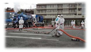
contamination density of the road surfaces within the difficult to return area is high (30,000 to 50,000 cpm). The pavement is furthermore the water permeable type, whereby contamination extends to the interior of the aggregate, thus lowering the effectiveness of the conventional high-pressure water.
