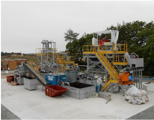
Fig. 1 Soil decontamination demonstration plant
