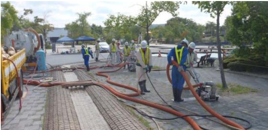
Fig. 1 A three-fold improvement in work efficiency was observed when using three cleaners for decontamination at the same time
