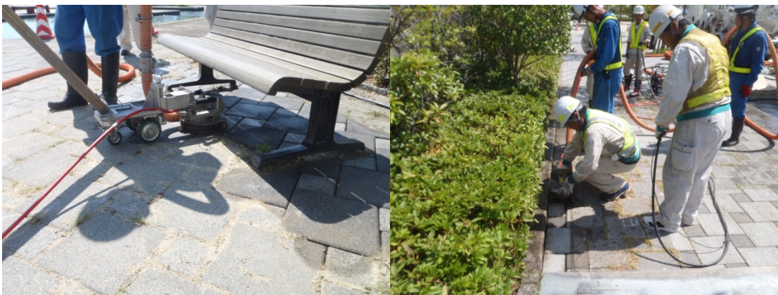
Fig. 2 Development of compact ultra-high pressure cleaners used for cleaning places under benches and corners that could not be decontaminated by existing cleaners.
